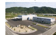
Kumayama Factory (Left: Plant building / Right: Office building and research laboratory)
